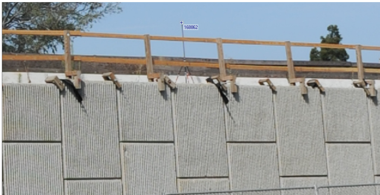
Figure 7: Reference target placed over survey location on top of wall
